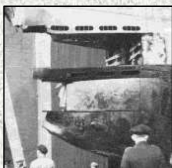
Above (B62): A somewhat damaged U 67 in October 1941. While some vents have been lost due to damage to the bow, this boat had port pattern A which was commonplace at the time. Above right (B63): The museum boat U 505, which presently has port pattern E, originally had port pattern B. Pattern E is unique, being formed due to years of corrosion in Chicago which resulted in one vent being covered over.
