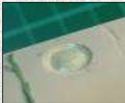
Above left (H15): The pilot holes for the round shaped covers.
