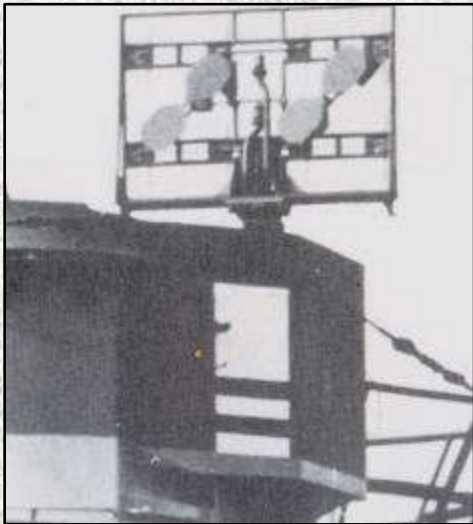
Left (C44): The FuMO 30 antenna raised above the purpose-built box on the port side of the tower.
